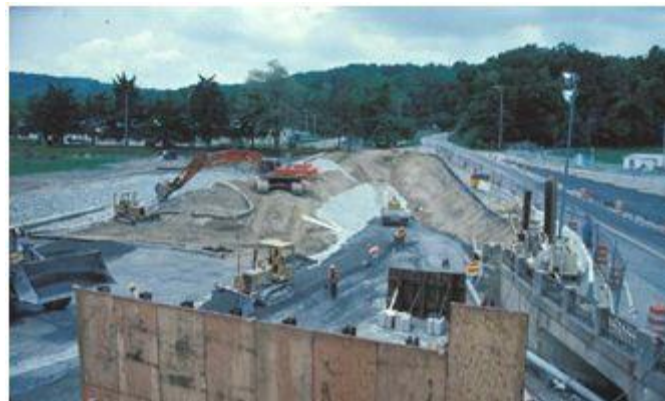
Figure 10. RCC construction at Lower Lake Royer Dam (provided by Maryland Department of the Environment).
