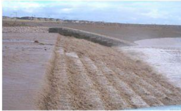
Figure 16. 2004 storm overflow at Red Rock Detention Basin Spillway (provided by Clark County Regional Flood Control District).
