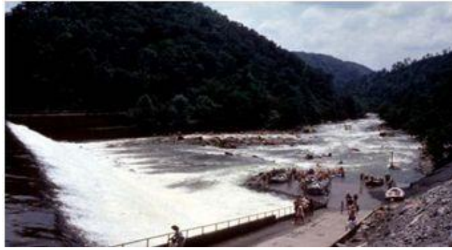
Figure 4. Close-up of Ocoee Dam No. 2 operating with rafts downstream.
