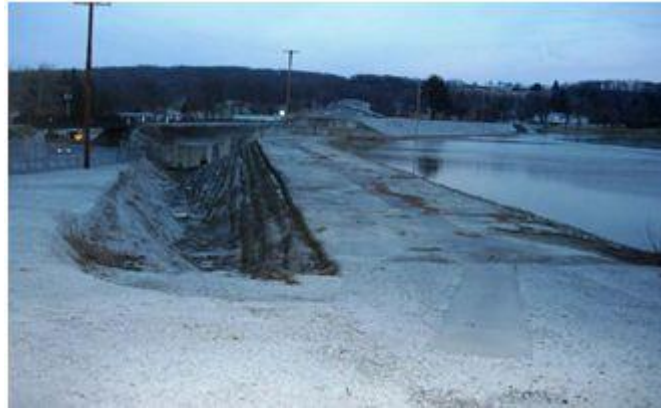
Figure 11. Lower Lake Royer Dam after 10 years of service.
