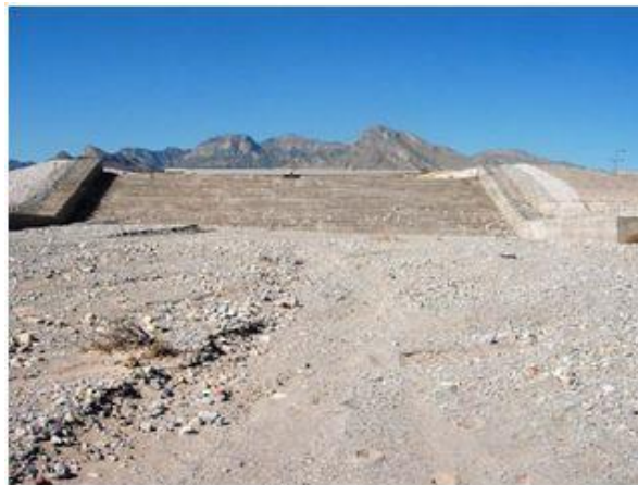
Figure 17. Red Rock RCC inflow spillway (February 2006).
