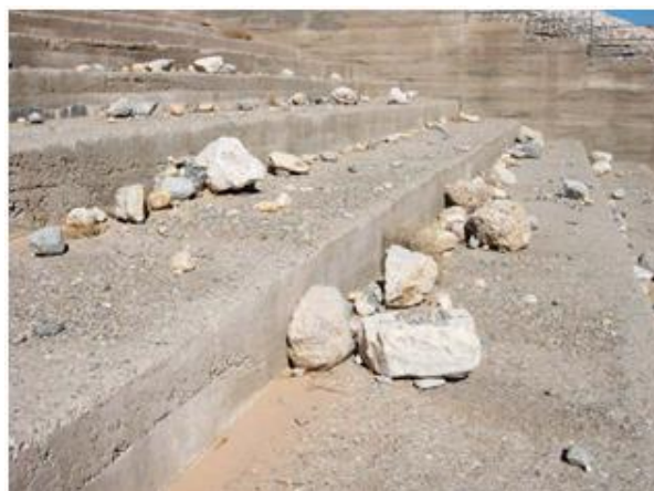
Figure 18. Boulders deposited on the RCC steps during 2005 storm. Photo taken in February 2006. Note limited wear of RCC step
