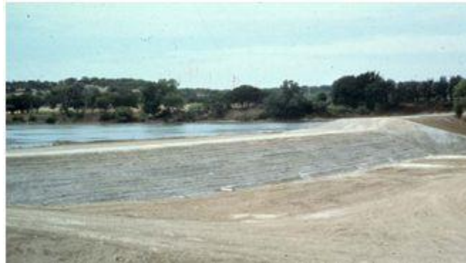
Figure 7. Brownwood Country Club Dam.
