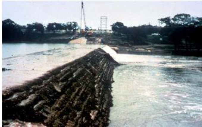
Figure 9. Kerrville Dam after major overtopping events.
