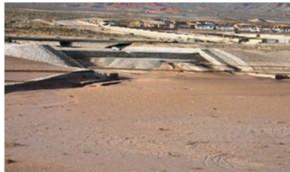
Figure 15. Red Rock RCC inflow spillway (January 2005). Note pile of sediment in stilling basin.
