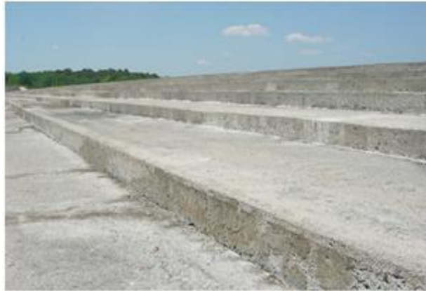
Figure 14. Excellent condition of RCC steps at Tholocco Lake Dam (May 2007).
