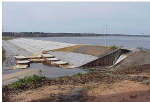
Figure 12. A view of principal and auxiliary spillways at Lake Tholocco Dam.
