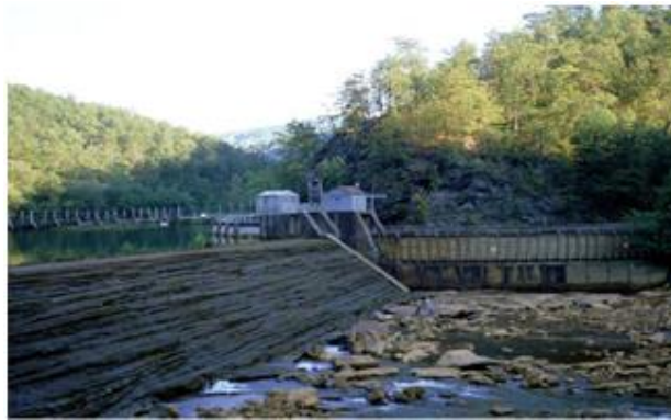
Figure 5. Ocoee Dam No. 2 after 27 years of service (provided by TVA).
